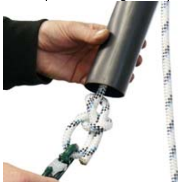
Figure 14: Rope fixing installation
